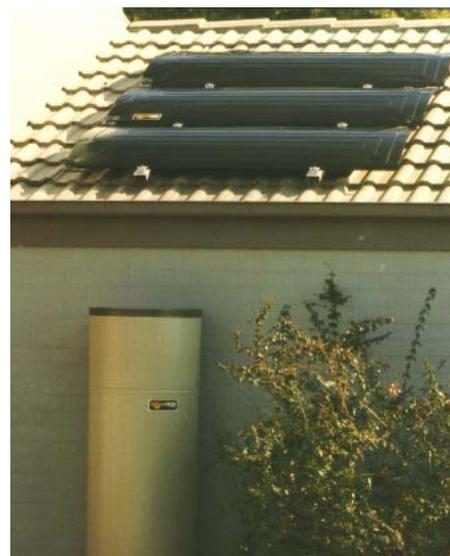
Solar boosted system with evaporator on the roof.
